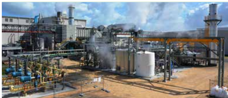
Kimberly-Clark Australia's $33 million cogeneration facility at Millicent Mill in South Australia.
