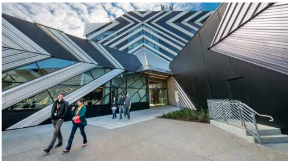
The New Horizons Building at Monash University. Source: Monash University
