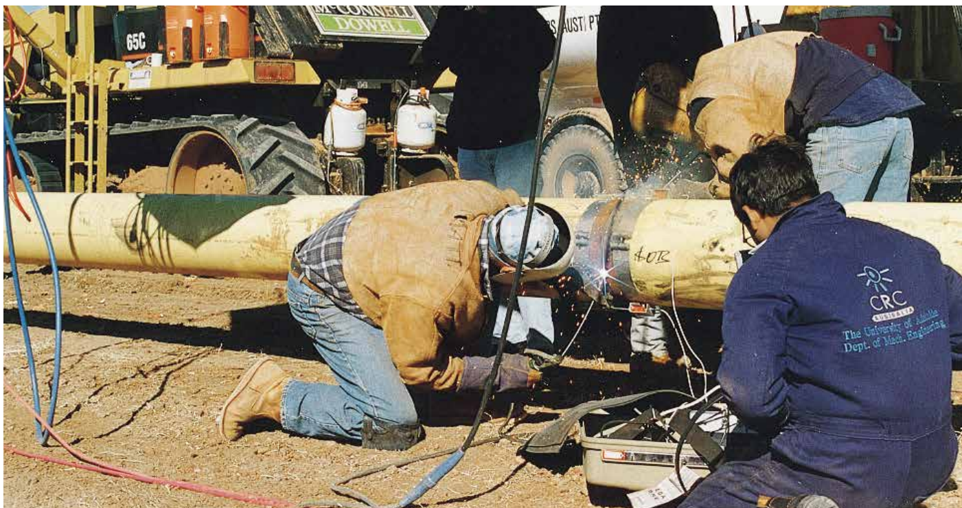
CRC-WS sponsored research and demonstration of the welding of X80 thin-walled pipe.
