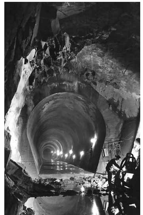
Welding for the iconic Snowy Mountains Hydro-Electric Scheme.
